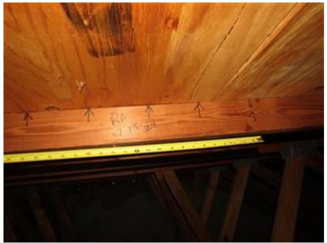
Roof to Deck Connection
