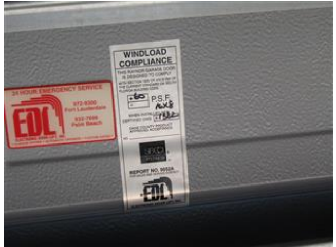
Hurricane Garage Door Verification
