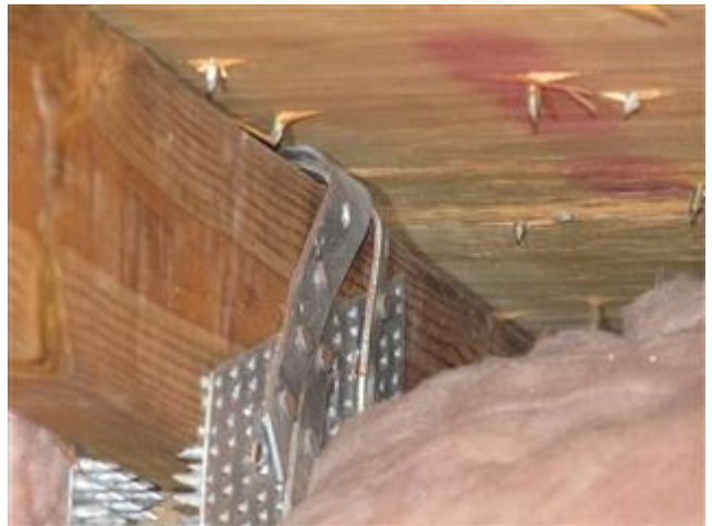
Roof to Wall Connection - Double Straps (Backside)
