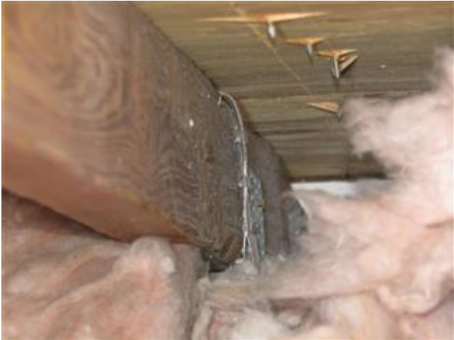
Roof to Wall Connection - Double Straps
