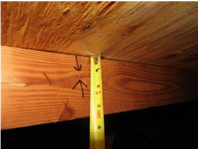
Roof to Deck Connection - 8D Nailing
