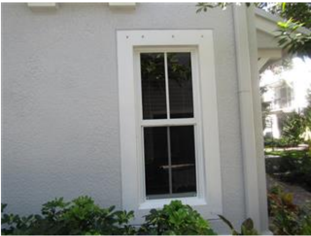
Hurricane Shutter Hardware Verification - Window and Glass Doors
