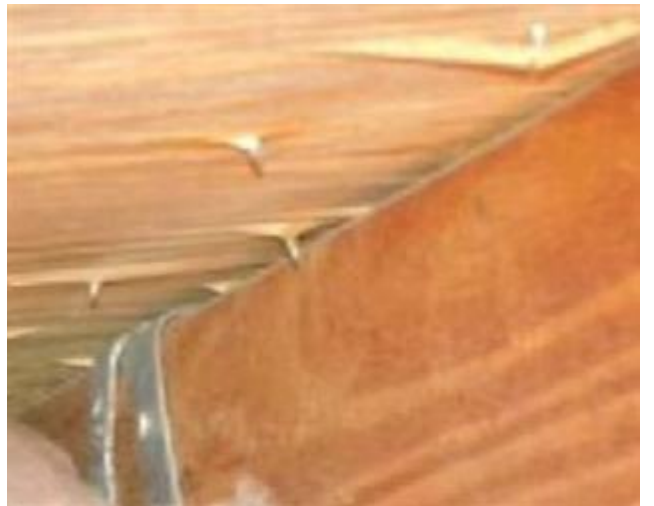
Roof to Wall Connection - Double Straps (Backside)
