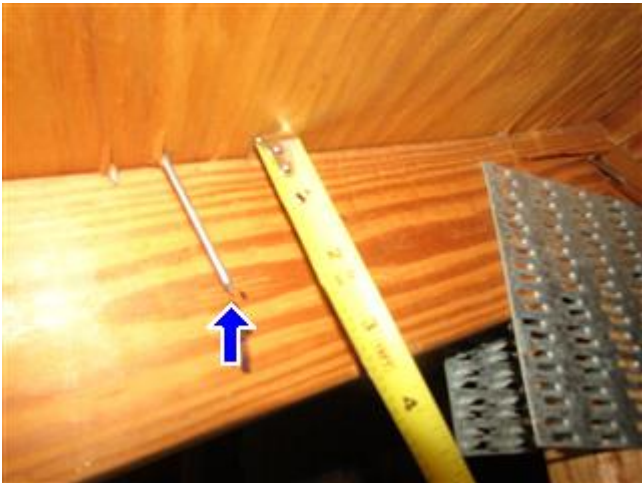
Roof to Deck Connection - 8D Nailing
