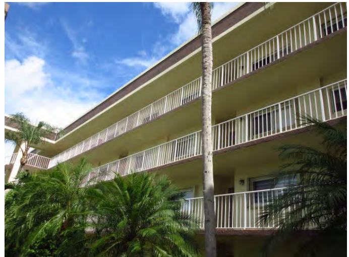
GENERAL VIEW OF BUILDING EXTERIOR FINISHES
