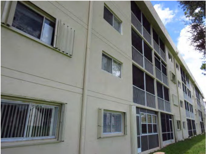
VIEW OF BUILDING EXTERIOR FINISHES
