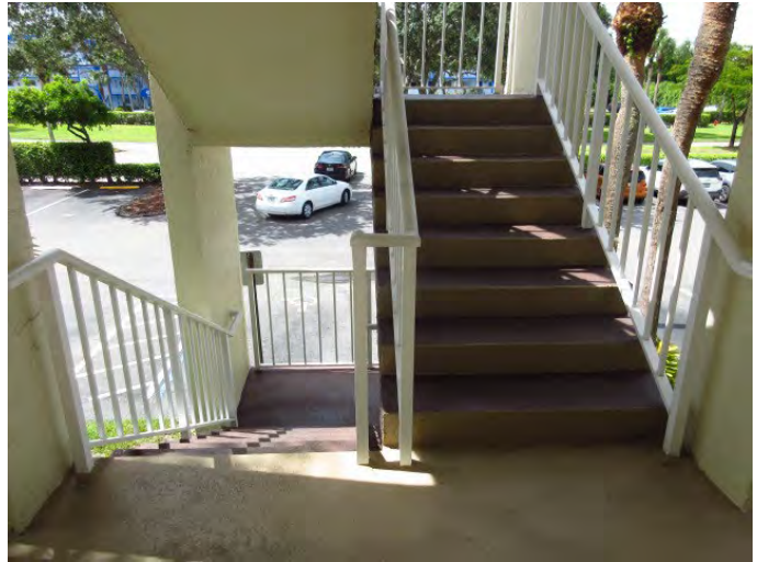
VIEW OF EXTERIOR STAIRS
