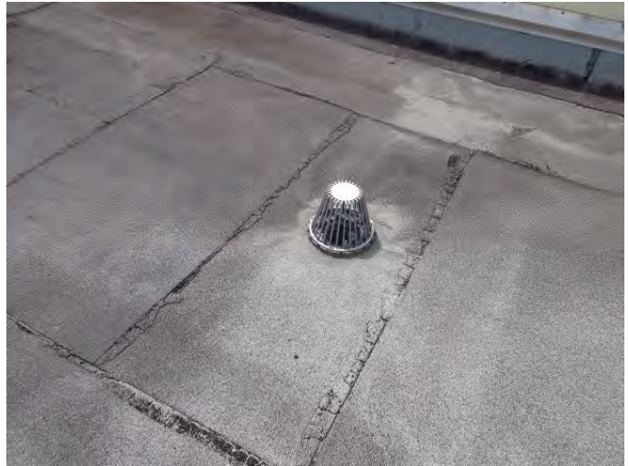
VIEW OF ROOF DRAIN
