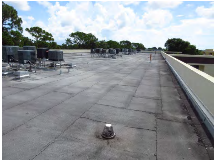
VIEW OF ROOF COVERING
