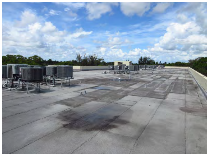
GENERAL VIEW OF ROOF COVERING
