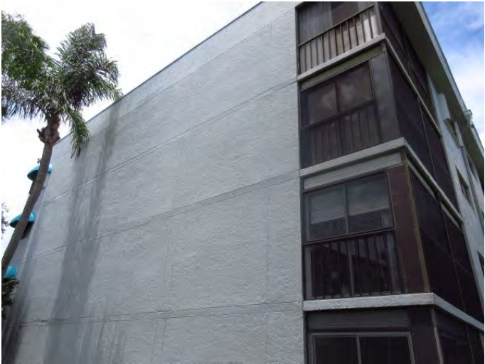
VIEW OF BUILDING EXTERIOR FINISHES
