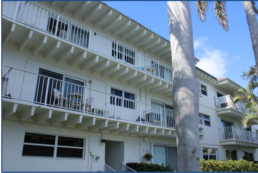
Photograph No. 3: Northern elevation
