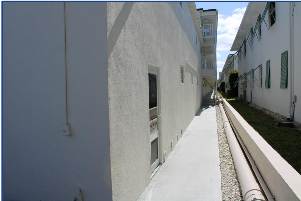
Photograph No. 4: Southern elevation
