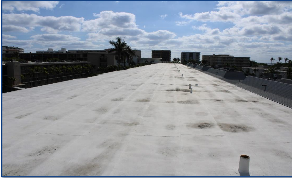
Photograph No. 27: Roof over units.
