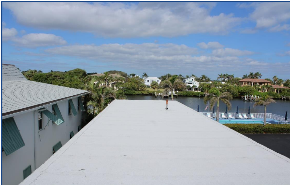
Photograph No. 28: Roof over laundry and storage area.
