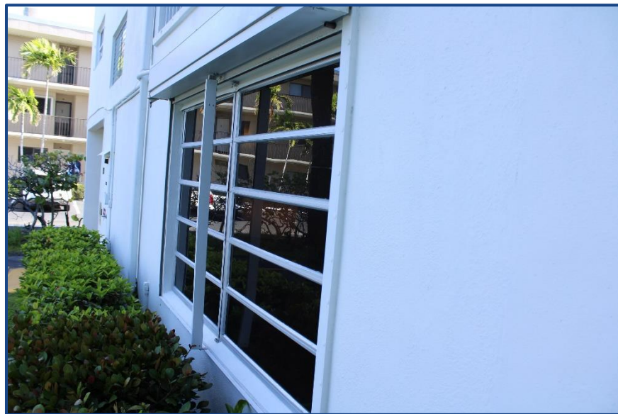
Photograph No. 30: Exterior window at common areas, typical.
