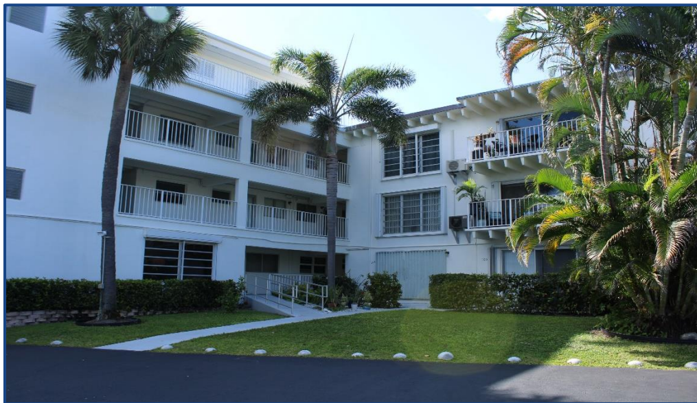
Photograph No. 6: Northern elevation
