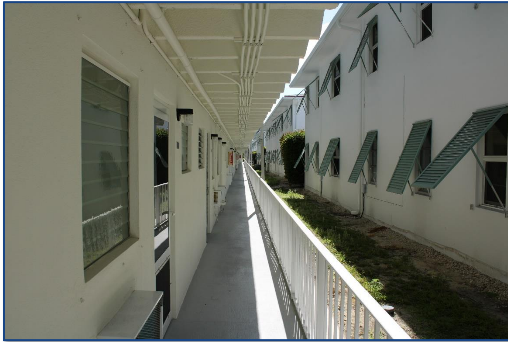
Photograph No. 23: Typical catwalk.
