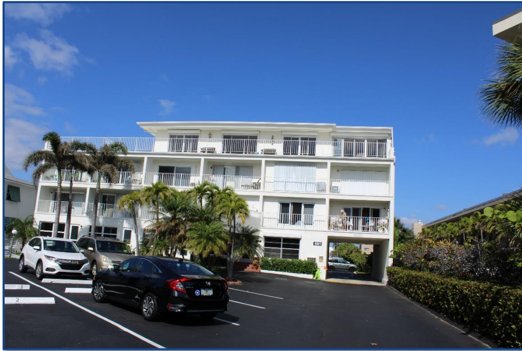
Photograph No. 1: East elevation
