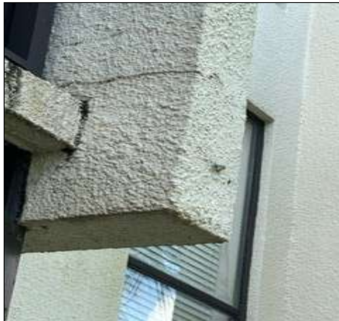
WALL REPAIR UNIT 201 ( EAST & NORTH SIDES )
