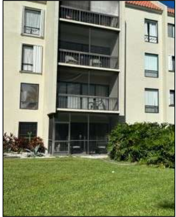
STACK #2 EAST ELEVATION
