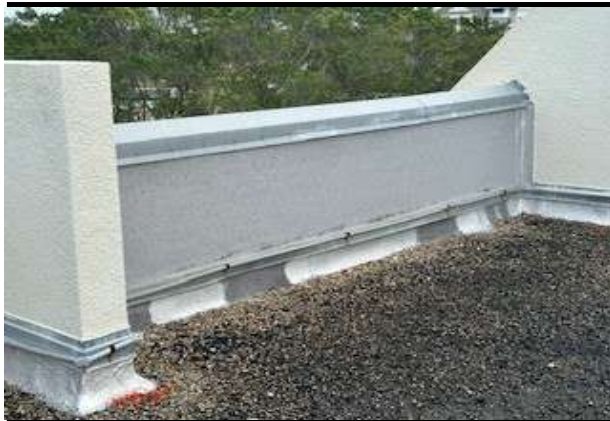
TYPICAL PARAPET WALLS BETWEEN MANSARD ENCLOSURES
