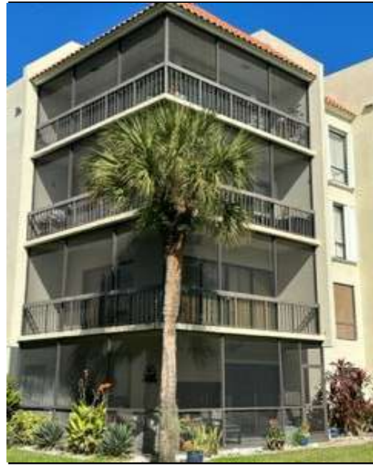
STACK #7 EAST ELEVATION
