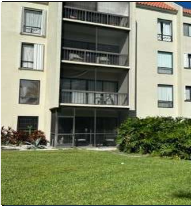
STACK #3 EAST ELEVATION
