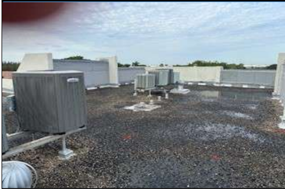
NORTH ROOF VIEW
