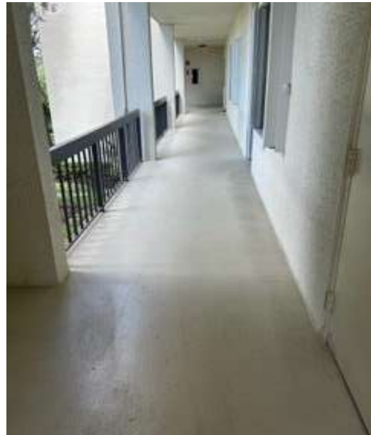
WALKWAYS - FLOORS 2 TO 4
