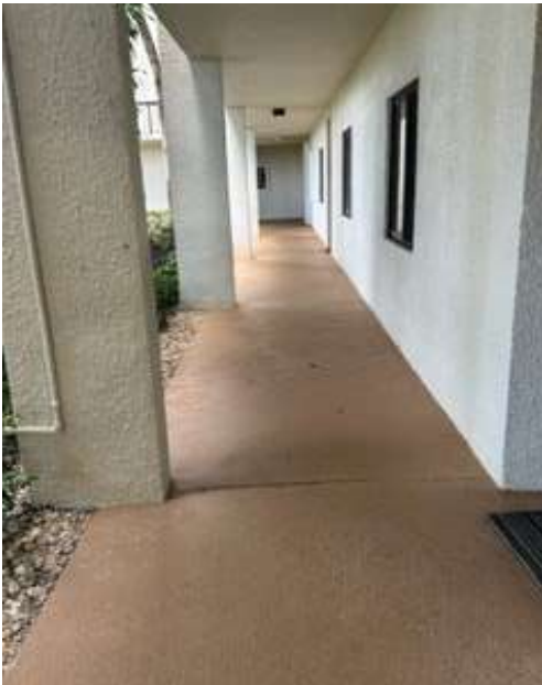
FIRST FLOOR WALKWAY
