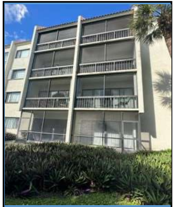
STACK #4 & 5 EAST ELEVATION
