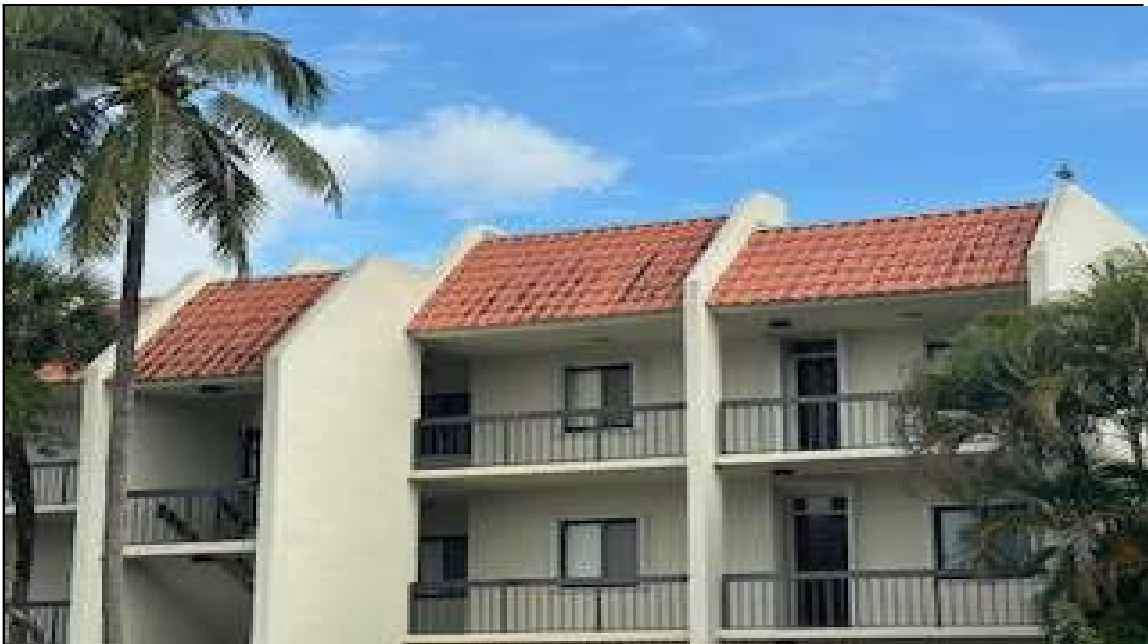
TYPICAL MANSARD TERRACOTTA /CLAY ROOFS
