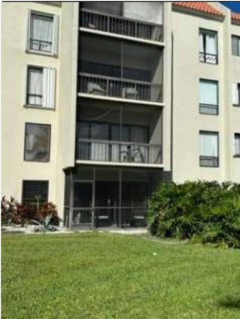
STACK #6 EAST ELEVATION
