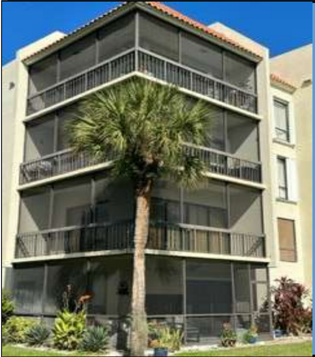
STACK #1 EAST ELEVATION
