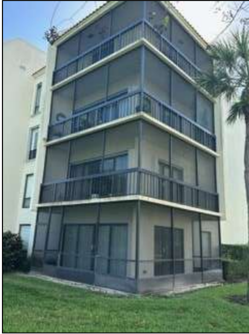
STACK #1 EAST ELEVATION
