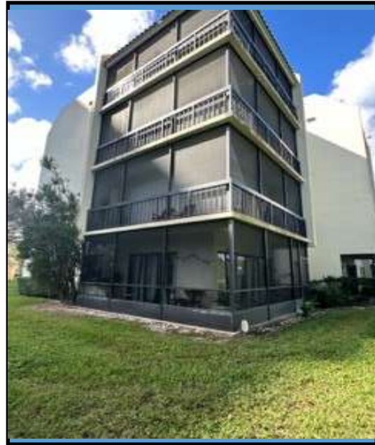
STACK #7 EAST ELEVATION
