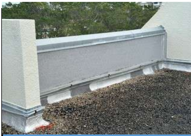
TYPICAL PARAPET WALLS BETWEEN MANSARD ENCLOSURES
