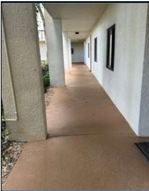
FIRST FLOOR WALKWAY
