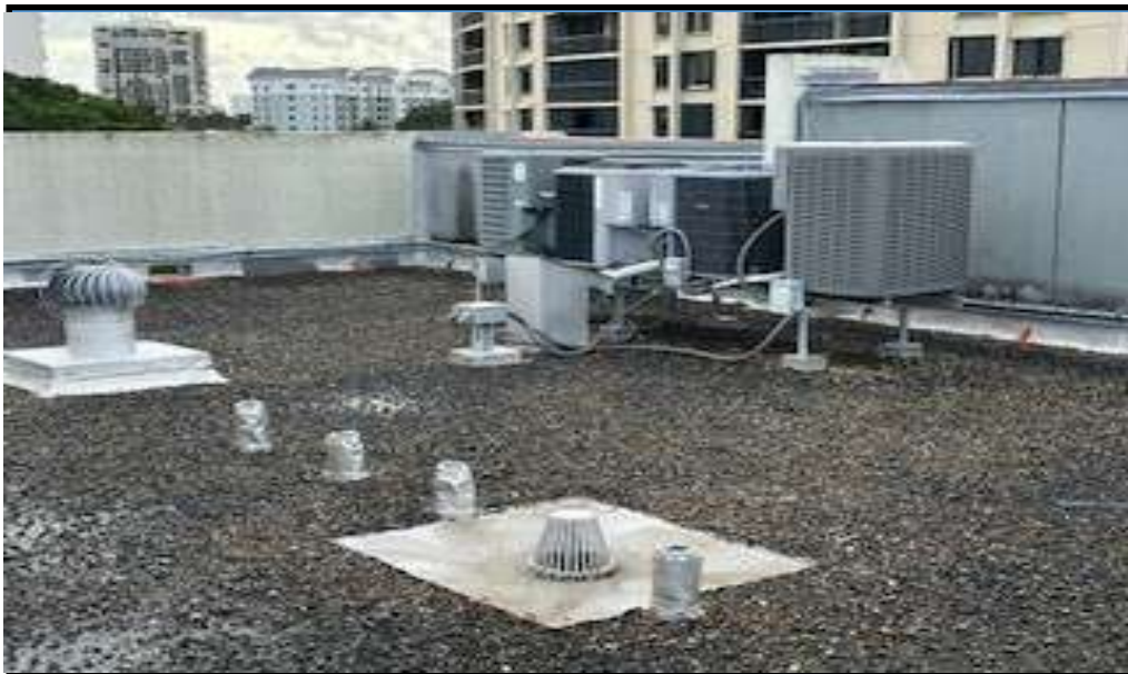
ROOF VENTS & A/C UNITS ON BUILT-UP GRAVEL ROOF
