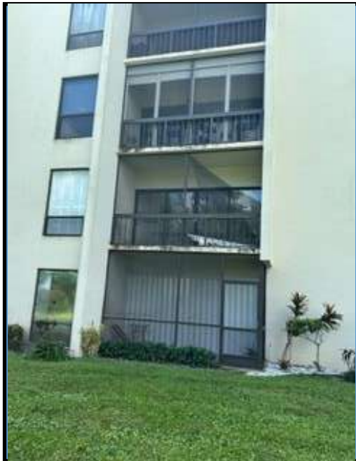
STACK #3 EAST ELEVATION
