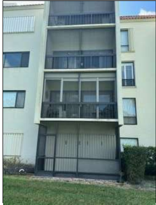
STACK #2 EAST ELEVATION
