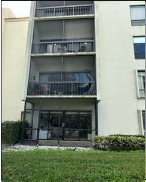
STACK #6 EAST ELEVATION
