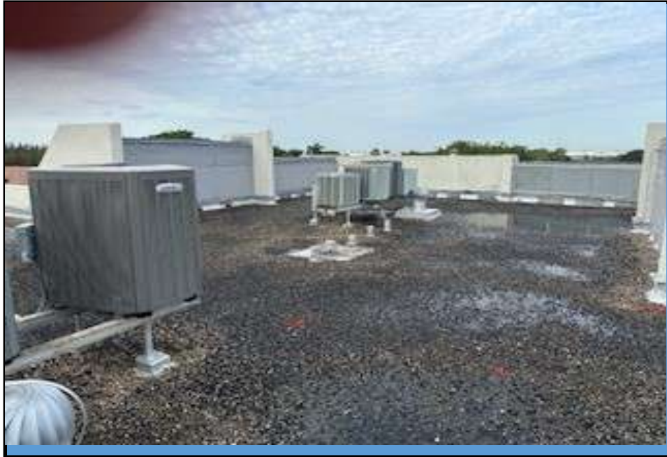
NORTH ROOF VIEW
