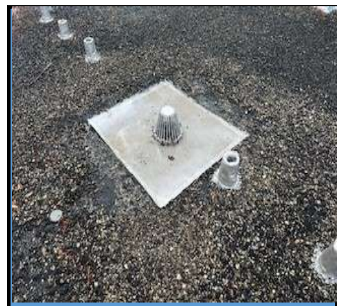
TYPICAL ROOF DRAIN
