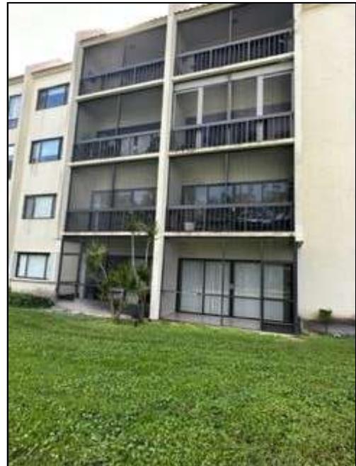
STACK #4 & 5 EAST ELEVATION
