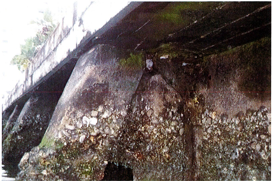
Photo 27: Photograph of a Complete Thru Crack of the Prestressed King Pile.
