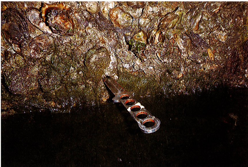
Photo 27: Photograph of a Significant Horizontal Crack in the Concrete Panel.
