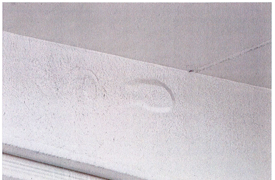
Photo 10: Photograph of a Concrete Spall/Deterioration on the side of the Concrete Supporting Structure.
