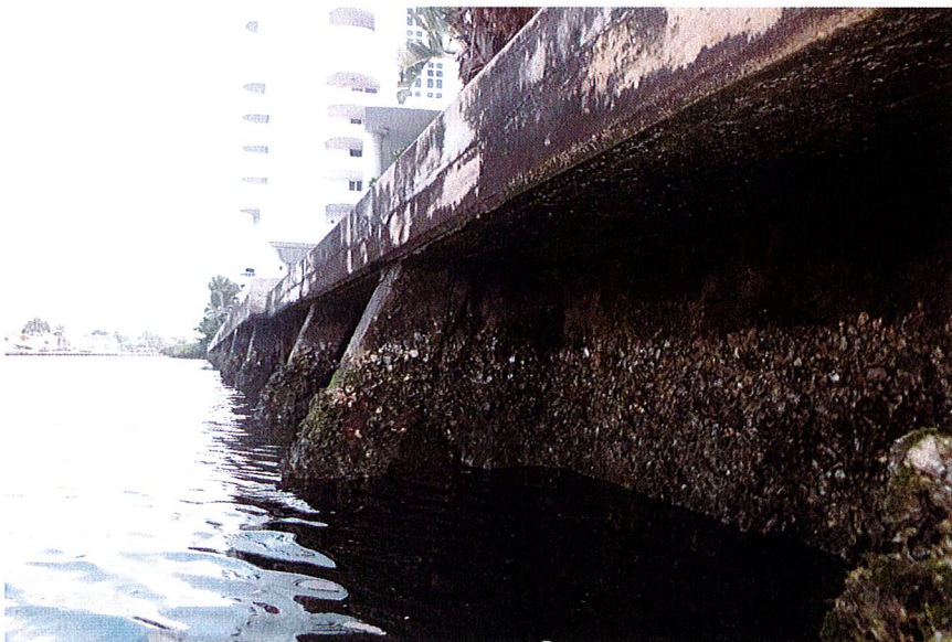
Photo 22: Photograph of the Seawall which Consist of Reinforced Concrete Panels, Prestressed King and Batter Piles, and a Reinforced Concrete Cap that Appears to have been Overlayed with a Secondary Pour.
