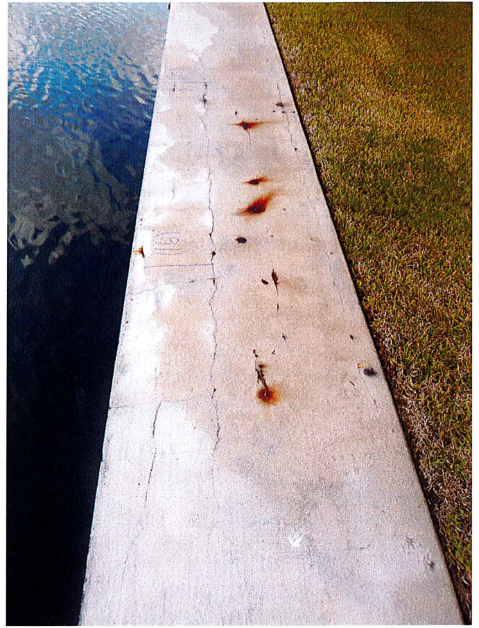
Photo 33: Deterioration of the Seawall Cap.
