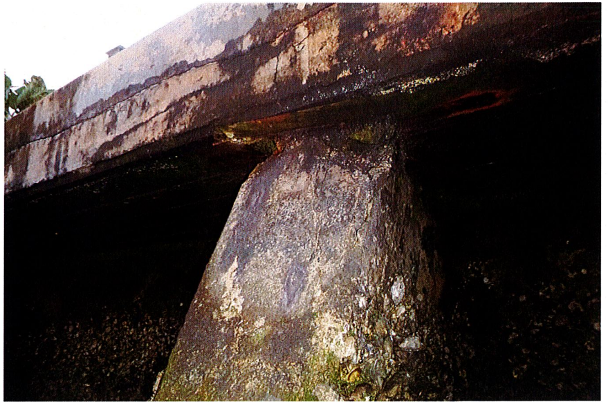
Photo 24: Photograph of the Cracking, Spalling, and Deterioation of the Reinforced and Prestressed Seawall Components.
