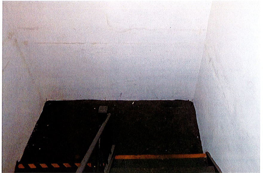
Photo 20: Photograph of the Staining of an Upper Level of the Stairwell Walls as a Result of Moisture Infiltration.
