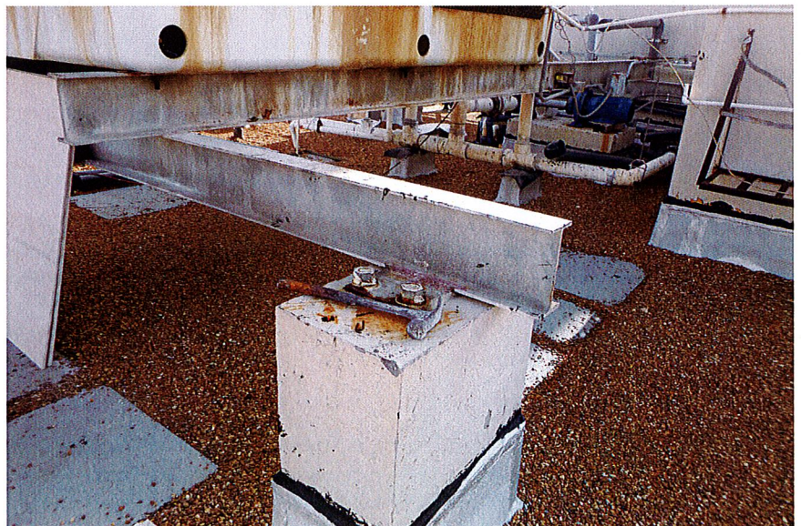
Photo 19: Close-Up Photograph of the Cooling Tower Steel I-Beam Support and Concrete Pedestals.
