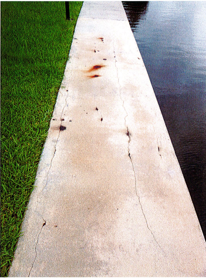
Photo 32: Deterioration of the Seawall Cap.
