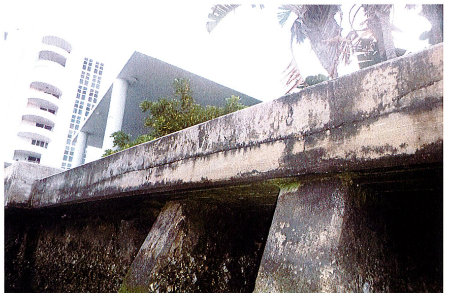
Photo 23: Close-Up Photograph of the Seawall Cap and the Continuous Crack along the Apparent Concrete Overlay.
