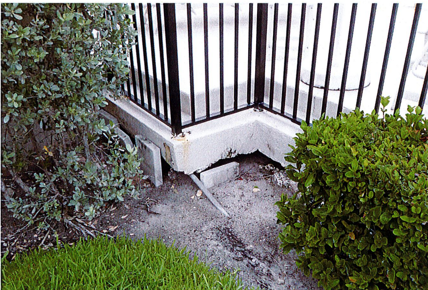
Photo 12: Photograph of the loss of Soil from Under the North Edge of the Concrete Pool Deck.
