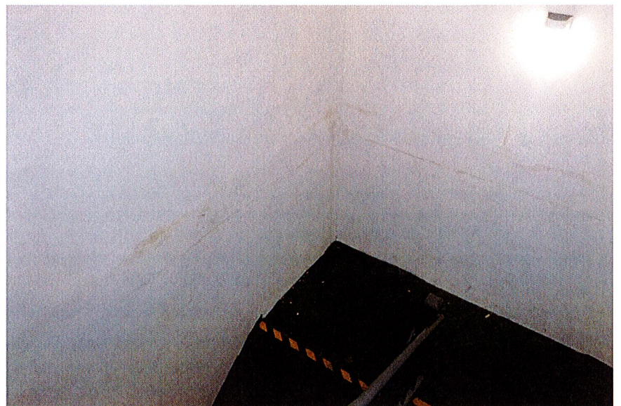
Photo 22: Photograph of the Staining of an Upper Level of the Stairwell Walls as a Result of Moisture Infiltration.
