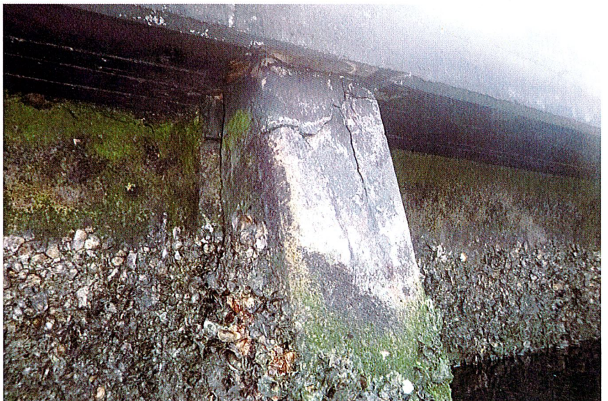
Photo 28: Photograph of the Cracking and Spalling of the Top of The Prestressed Concrete Batter Pile, Immediately underneath the Seawall Cap.
