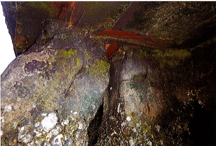
Photo 25: Close-Up Photograph of the Cracking, Spalling, and Deterioation of the Reinforced and Prestressed Seawall Components.
