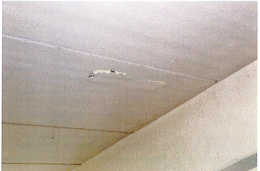
Photo 8: Photograph of the Typical Concrete Spall/Deterioration on the Undersided of a Prestressed Concrete Roof Panel.
