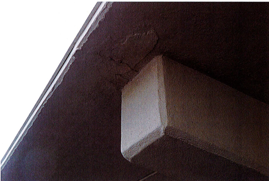
Photo 9: Photograph of a Typical Concrete Spall/Deterioration on the Underside of the Edge, Along the Intersection of the Prestressed Concrete Roof Panels.
