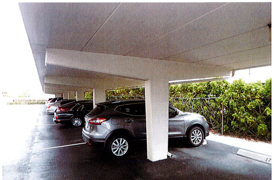
Photo 7: Close-up Photograph of the Typical Parking Structures which are comprised on Prestressed Concrete Roof Panels Supported by Concrete Support Structures.
