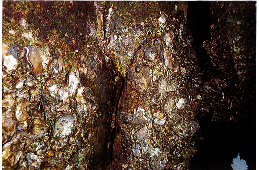
Photo 29: Close-Up Photograph of the Severe Cracking, Deterioration, and Deformation of the Prestressed Concrete Seawall Components.
