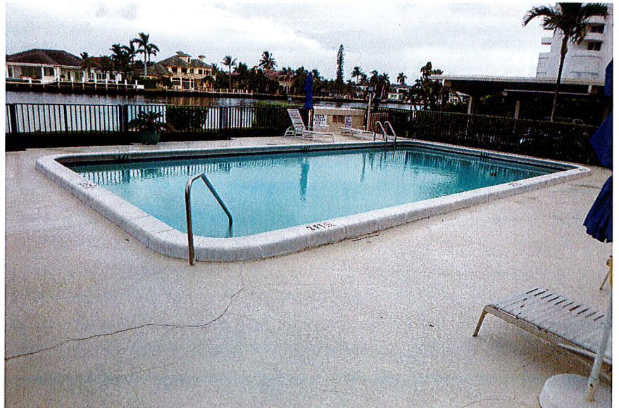
Photo 11: Photograph of the Typical Cracking of the Concrete Pool Deck.
