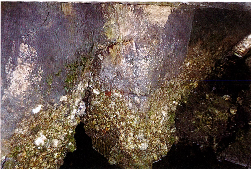
Photo 30: Close-Up Photograph of the Severe Cracking, Deterioration, and Deformation of the Prestressed Concrete Seawall Components.
