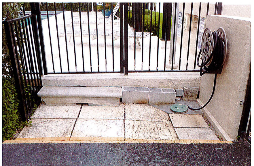
Photo 13: Photograph of the Placement of a concrete Step and Blocks to Cover the loss of Soil from Under the North Edge of the Concrete Pool Deck.
