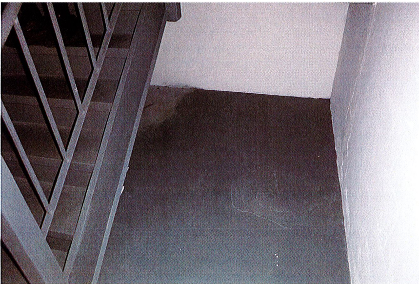
Photo 21: Photograph of the Staining of the Ground Floor of the Stairwell Walls as a Result of Moisture Infiltration.
