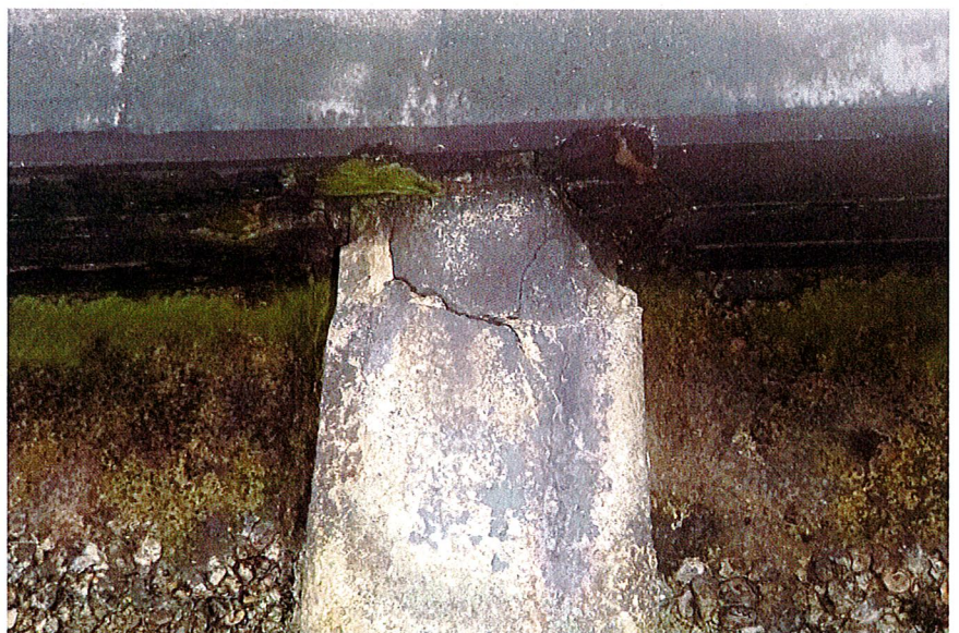
Photo 31: Photograph of the Cracking and Spalling of the Top of The Prestressed Concrete Batter Pile, Immediately underneath the Seawall Cap.
