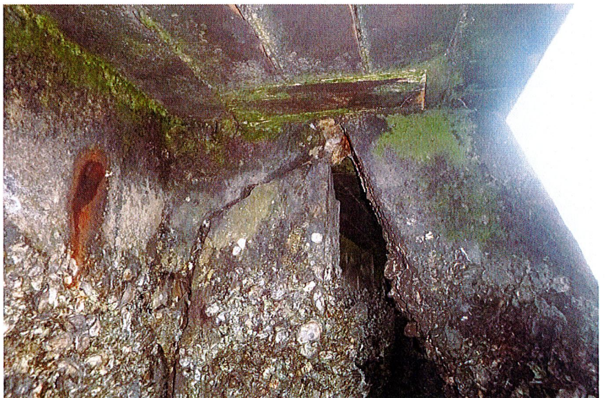
Photo 26: Photograph of a Complete Thru Crack of the Prestressed King Pile and Severe Oxidation of the Panel Tie-Back.
