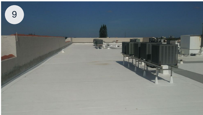
New GAF Single-ply TPO Roof
