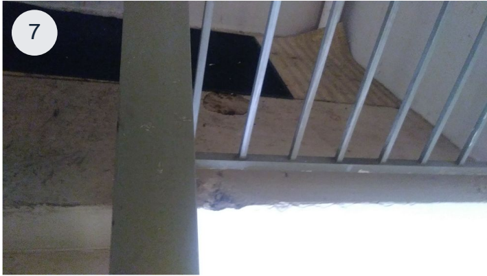
Reinforced Concrete deck
