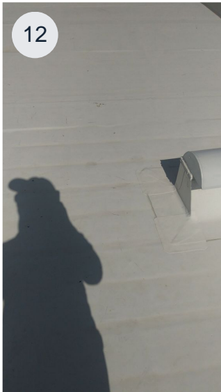
New GAF Single-ply TPO Roof
