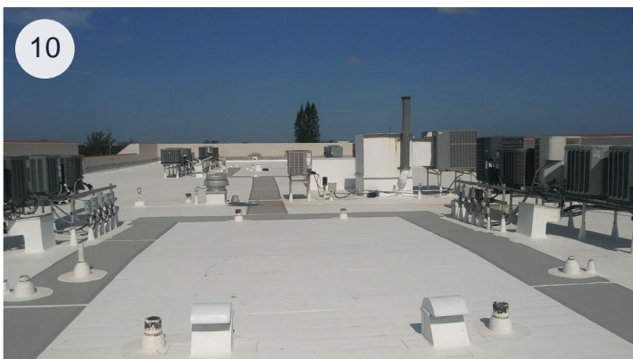
New GAF Single-ply TPO Roof
