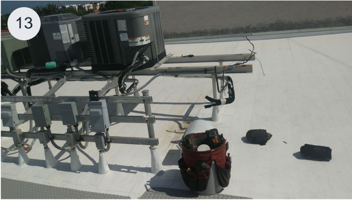
New GAF Single-ply TPO Roof
