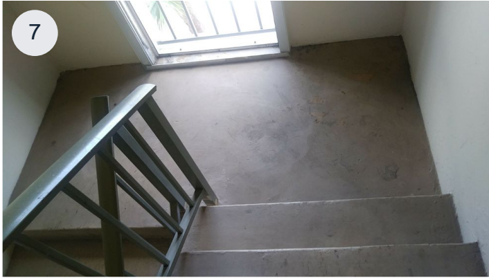
Reinforced concrete deck
