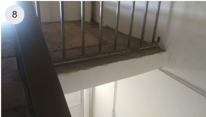
Reinforced Concrete deck
