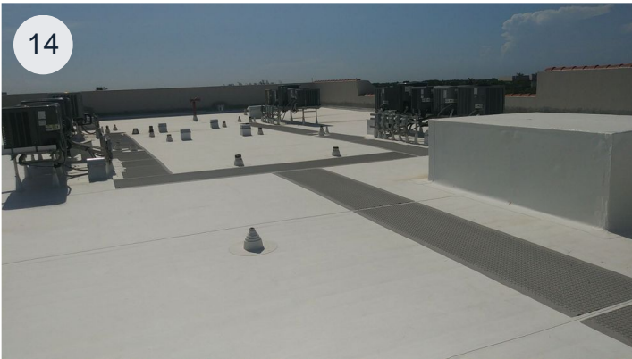
New GAF Single-ply TPO Roof
