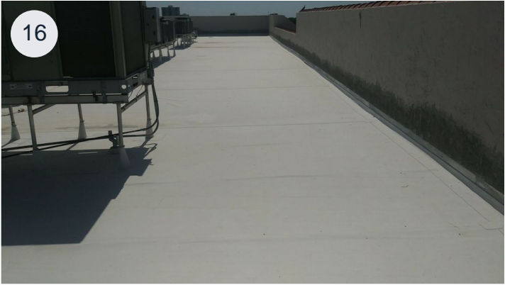
New GAF Single-ply TPO Roof
