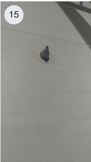
New GAF Single-ply TPO Roof
