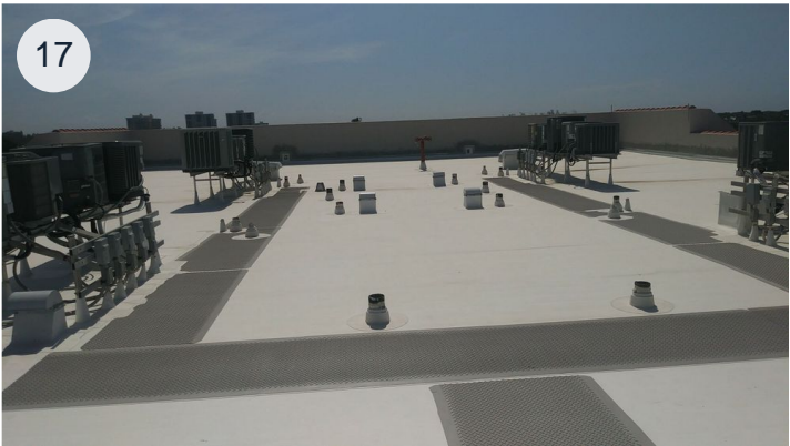
New GAF Single-ply TPO Roof
