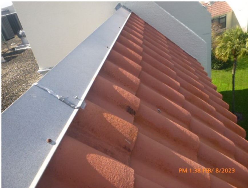
Built Up Tar & Gravel Roof Covering
