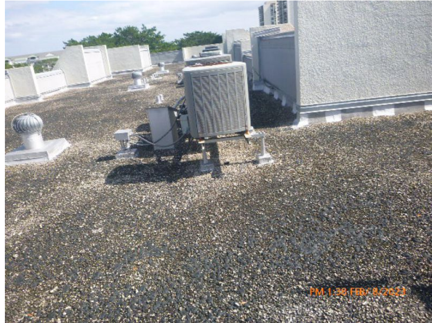
Built Up Tar & Gravel Roof Covering
